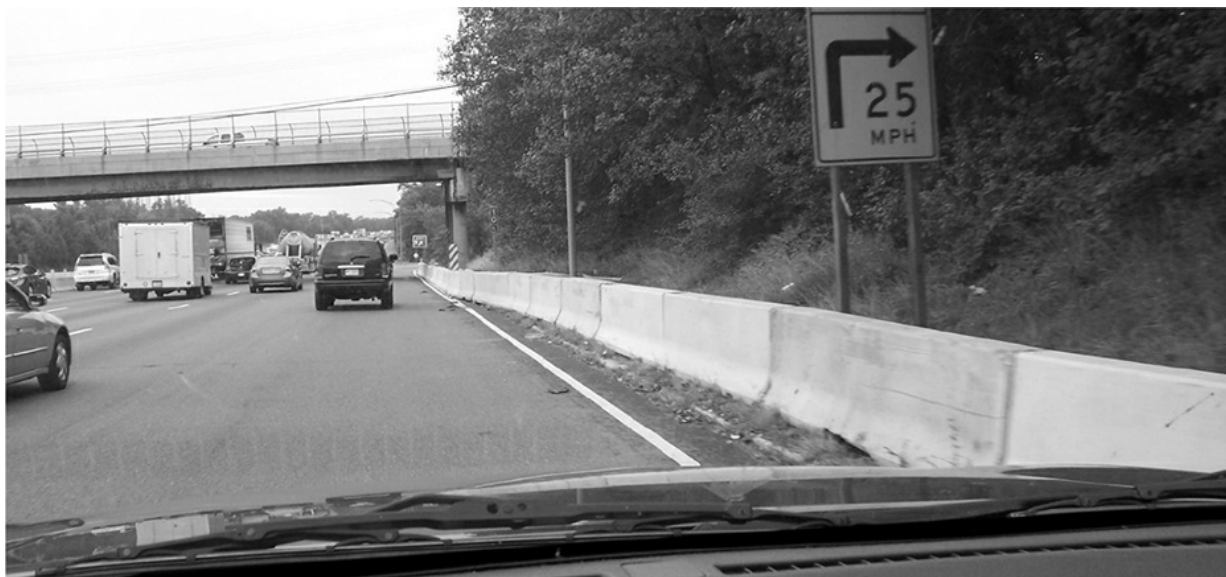
Figure 3-9: A Jersey barrier
